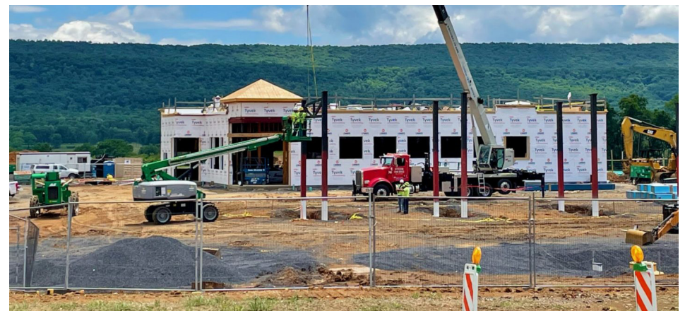
Sheetz on Whitehall Rd. under construction. Photo: Ben Jones, statecollege.com
