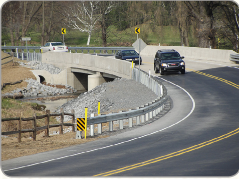
The State Route 3011 Branch Road Bridge was replaced in 2012. The rehabilitation and replacement of structurally-deficient bridges is a primary focus of state and local officials.
