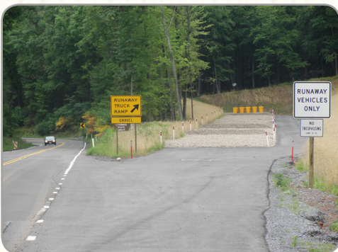
The Route 26 truck pull-off and escape ramp on Pine Grove Mountain were constructed in 2012. Projects such as these are important to improving safety and preserving the existing road system in the Centre Region.
