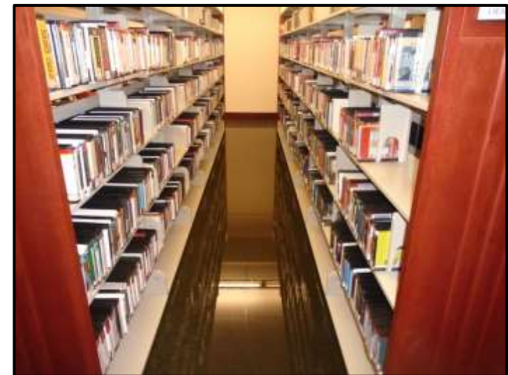
Figure 53. Over $50,000 of drywall damage and damaged books and audiobooks was sustained in the flood and reimbursed by insurance.
